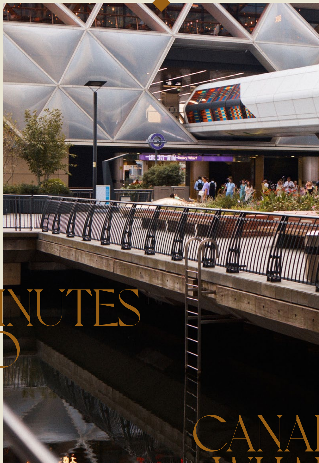
CROSSRAIL PLACE Canary Wharf's iconic Elizabeth line station
